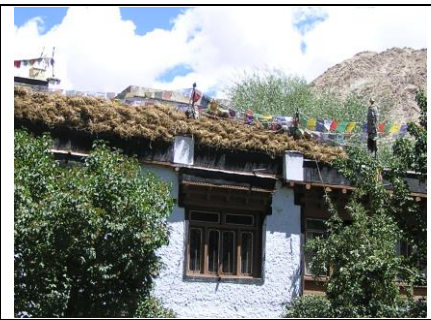
Insulated roof top
